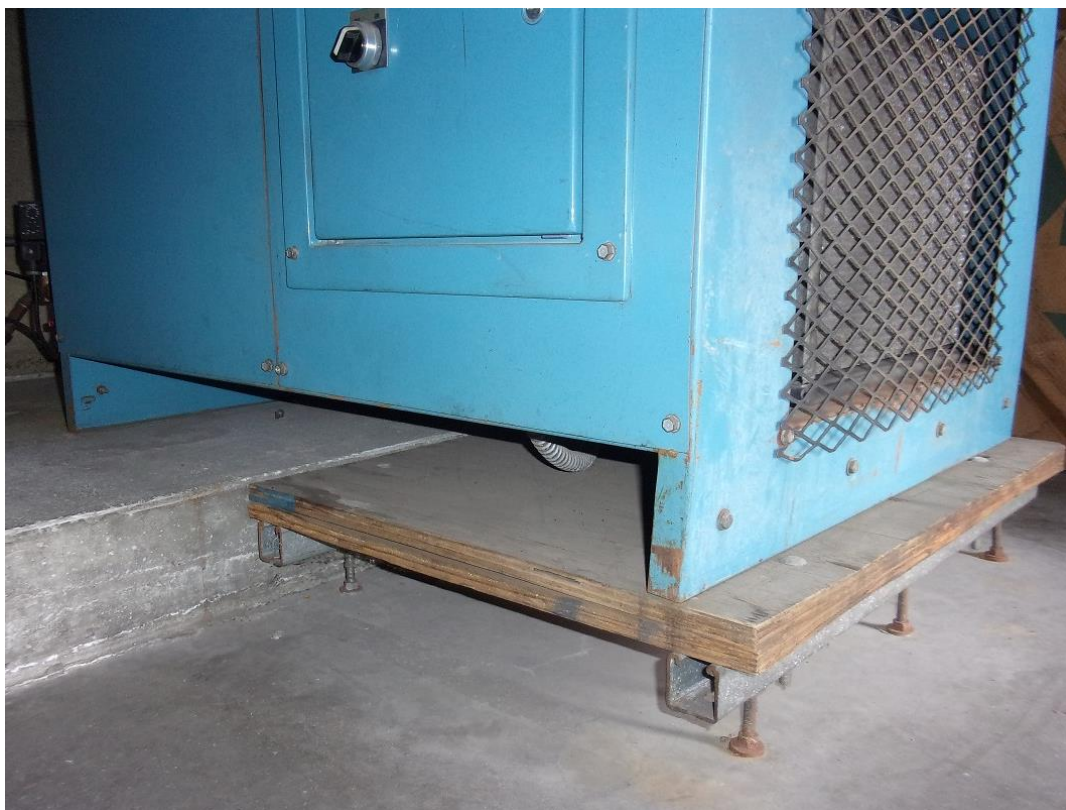
Figure 8: Air Dryer Support Platform (BASE BID)
