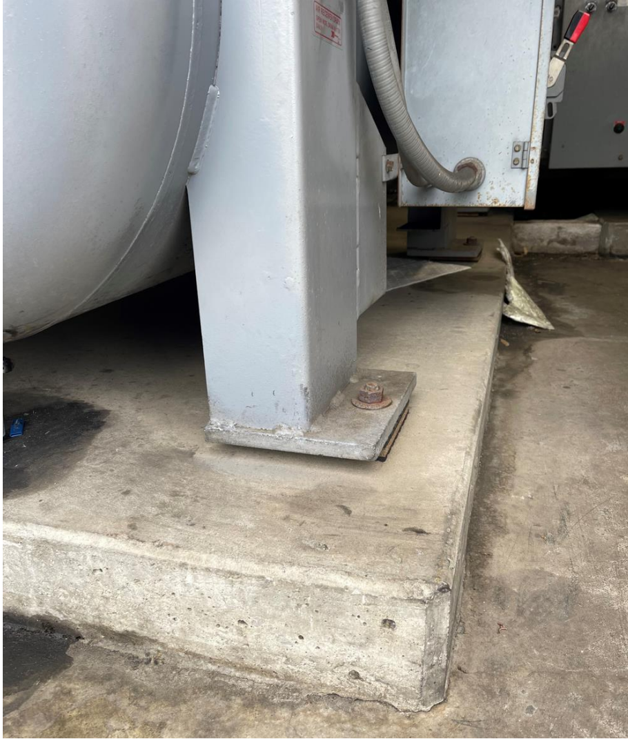
Figure 6: Compressor Mount & Foundation
