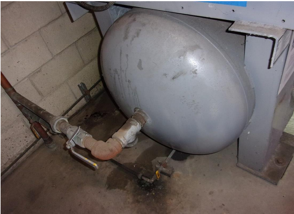
Figure 5B: Compressor 2 Outlet & Drain (BASE BID)
