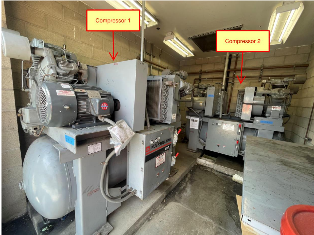
Figure 3: Compressor Room W/ Two Reciprocating Compressor (BASE BID)
