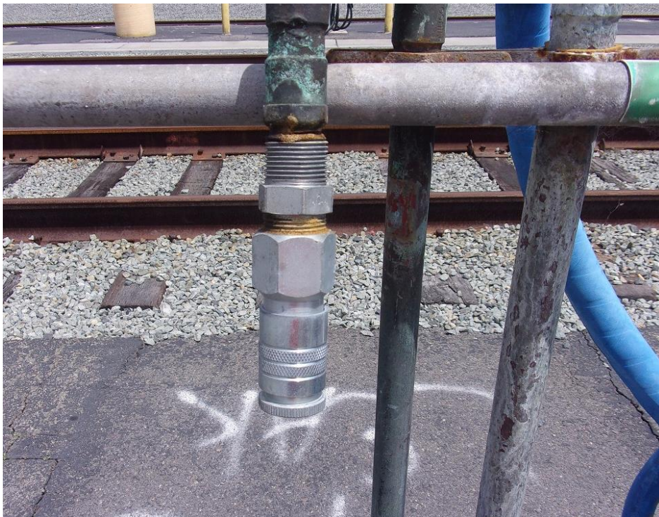
Figure 13: Close-Up of Current Quick Connect (BID OPTION 1)
